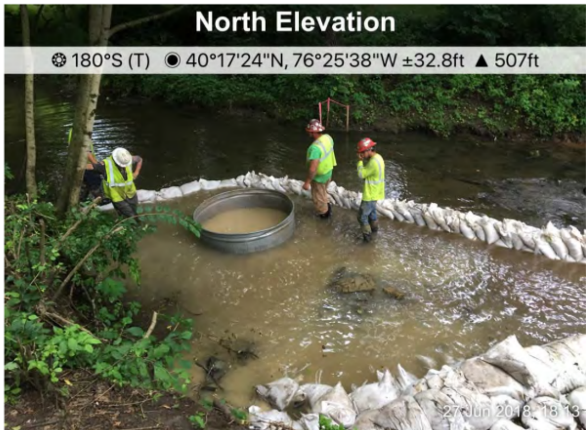
Photo taken by PG with GES, Inc. on June 27, 2018
