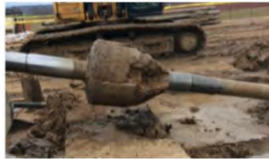
Balled Up Reamer April 3, 2017
